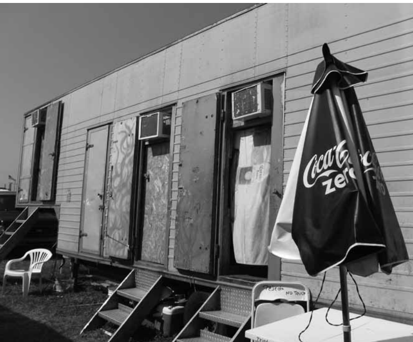
H-2B workers usually reside in employer-provided trailers on or near the fairgrounds. The trailers are often cramped, improperly maintained, and infested by roaches and bed bugs. Photo: Carson Osberg
